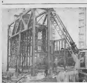
The new preheat furnace for the Cat Cracker takes shape.
